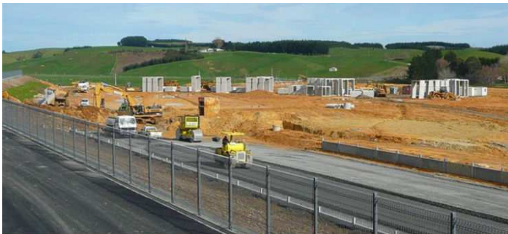
Hampton Downs – Tunnel frames and Pit area
