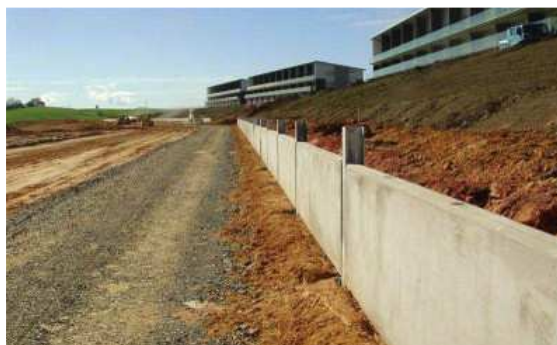
Construction of Front Straight barriers and track at Hampton Downs - May 09
