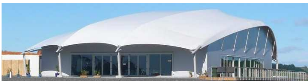
The new Hamptons Convention/Events centre located in the Pit Paddock at Hampton Downs Motorsport Park
